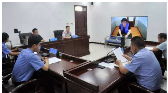
Tiandy's integrated video technology prosecutorial interrogation system installed in Nanyang City, Henan Province, in 2021. Source: Tiandy.
